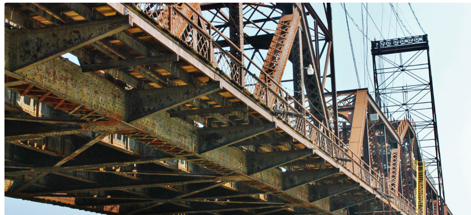
▼ Livingston Avenue Bridge
