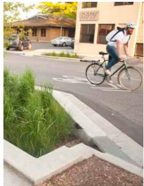
Figure 25. Small scale rain garden design as part of the Portland Green Streets program.
