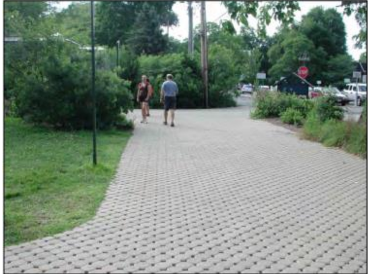
Figure 12. Walkway with permeable pavers in Hudson Park, Cold Spring NY. Courtesy of NYSDEC.
