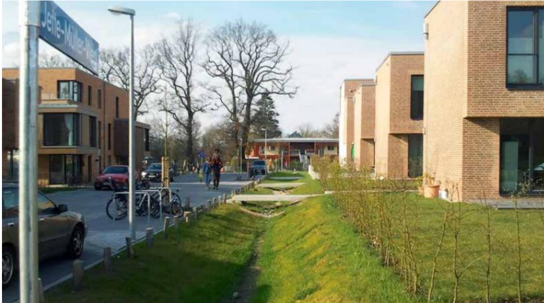
Figure 24. Hamburg street side ditch features address urban flooding.
