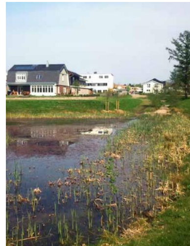
Figure 23. Wet basins collect and detain runoff after heavy rainfall events.
