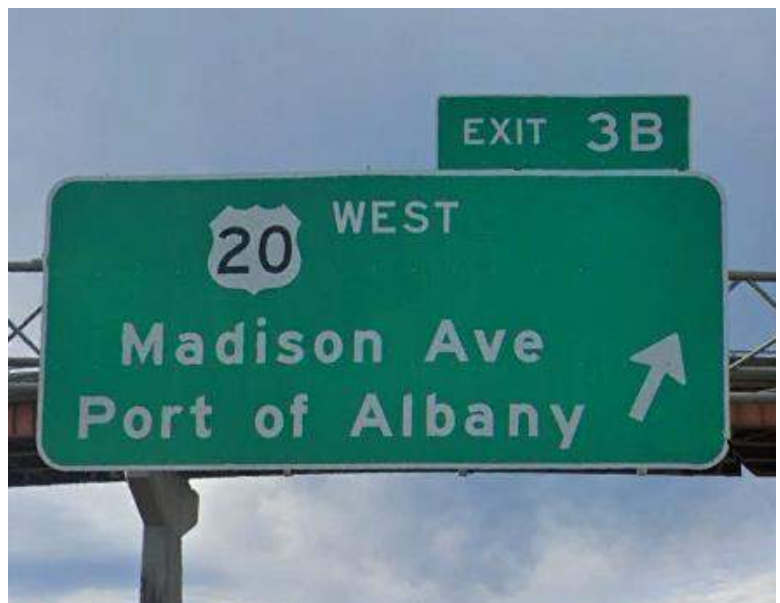
Example of Exit 3B sign that will need replacement
