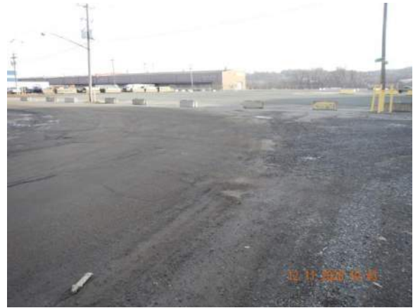
Smith Blvd/Raft St
