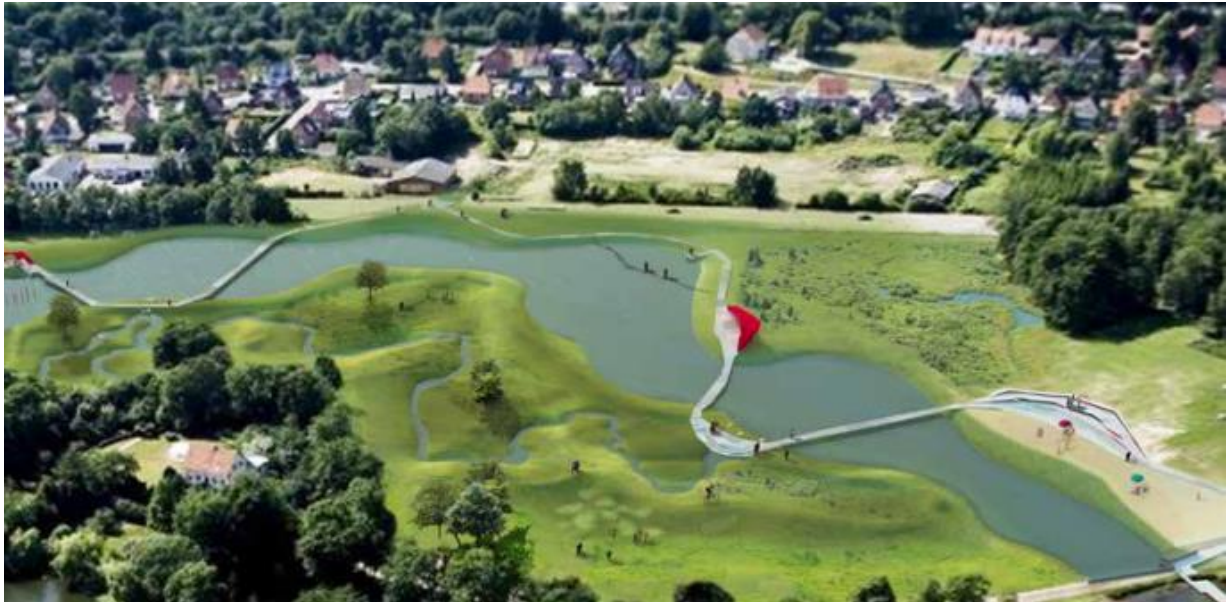
Figure 28. Large scale retention areas in Copenhagen manage coastal and precipitation based flood risks.
