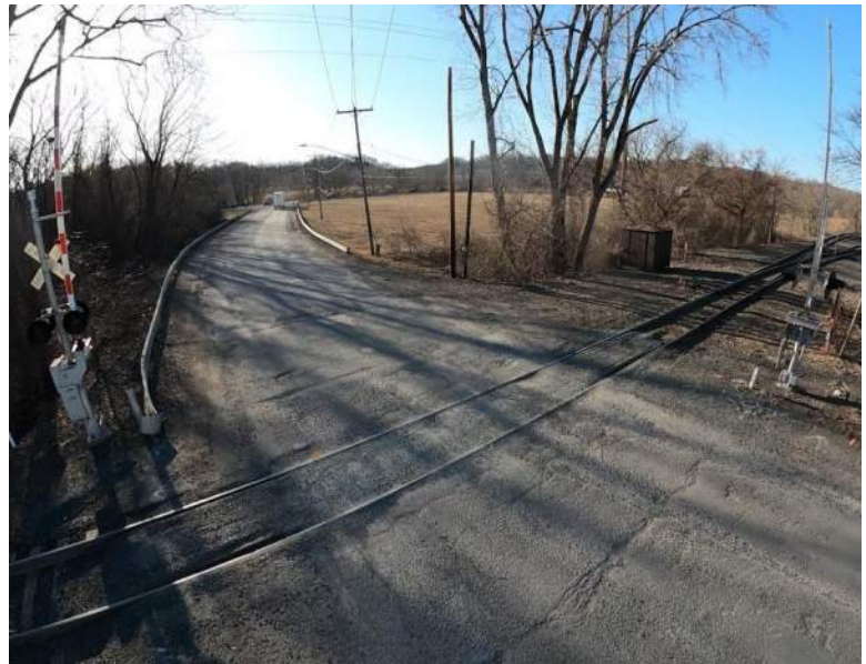
S. Port Rd Highway-Rail Crossing
